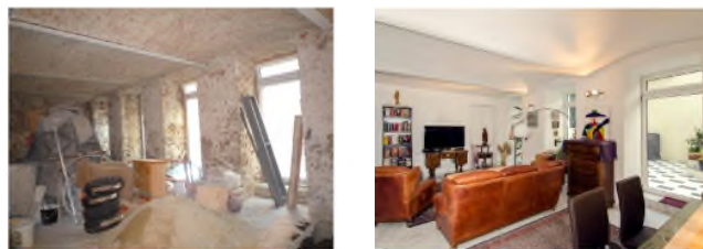
Figure 2: Example of a renovation using FRIDS
